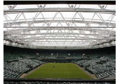
Wimbledon's Centre Court roof (Photo: Tommy Hindley)
