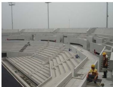
Beijing Olympic Tennis Centre under construction
